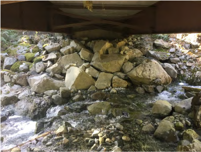
Right Bank Abutment when facing downstream
