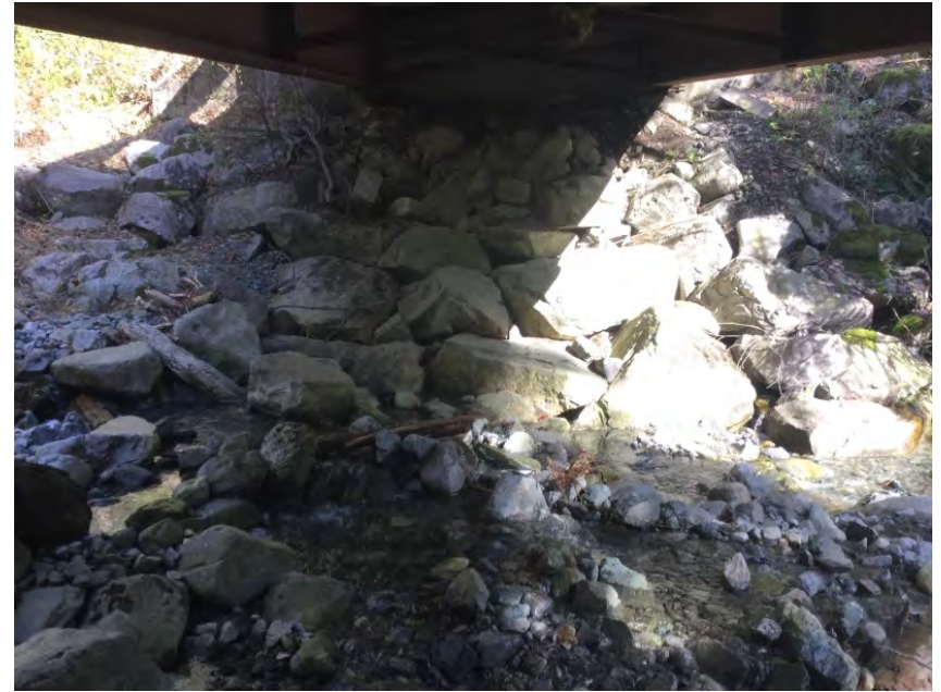
Left Bank Abutment when facing downstream
